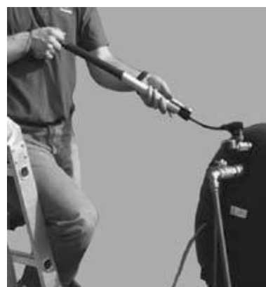
Figure 7.2 Pressurising the closed circuit
